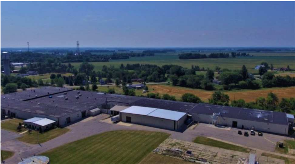
Trinity facilities, West Unity, OH
